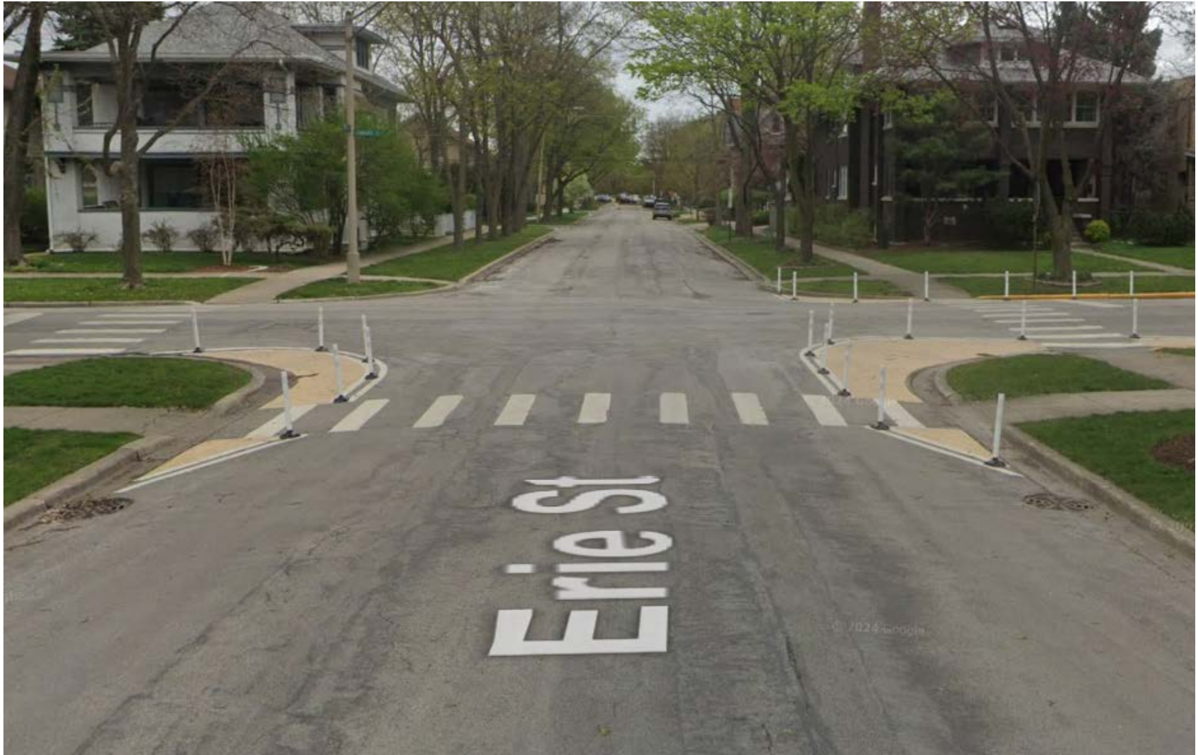
Paint and Post Curb Extension Example
